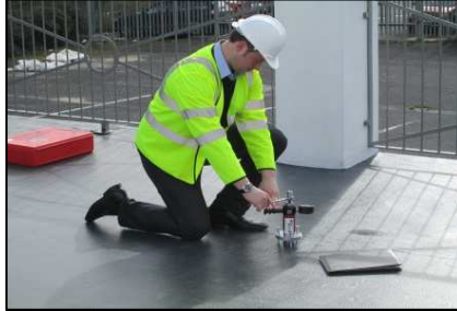
Substrate Pull-off Testing
