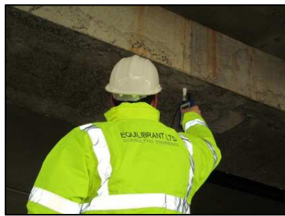
Concrete Inspection & Testing
